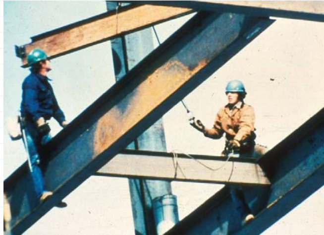
Assembling the structure of multi-storey building - connecting the secondary beams
