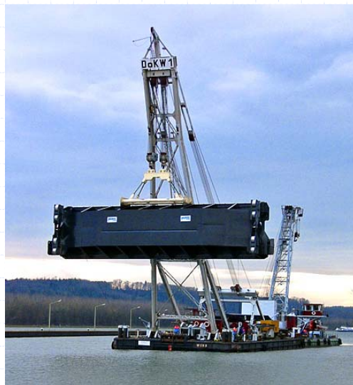
Lifting of the structure by floating crane
