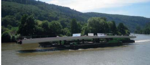
Transport of the Neckar Bridge on ship
