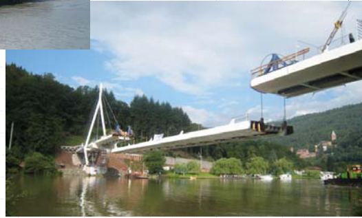
Assembling the Neckar Bridge Zwingenberg, Germany
