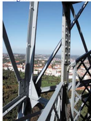
Riveted connection on Petřín tower
